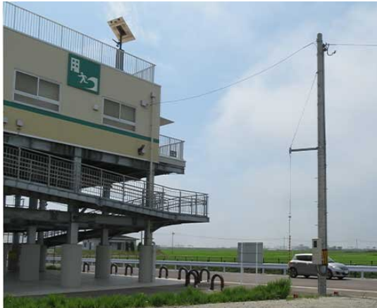
A tsunami evacuation tower designed after the experience of the Great East Japan Earthquake and Tsunami. Credit: Tohoku University
