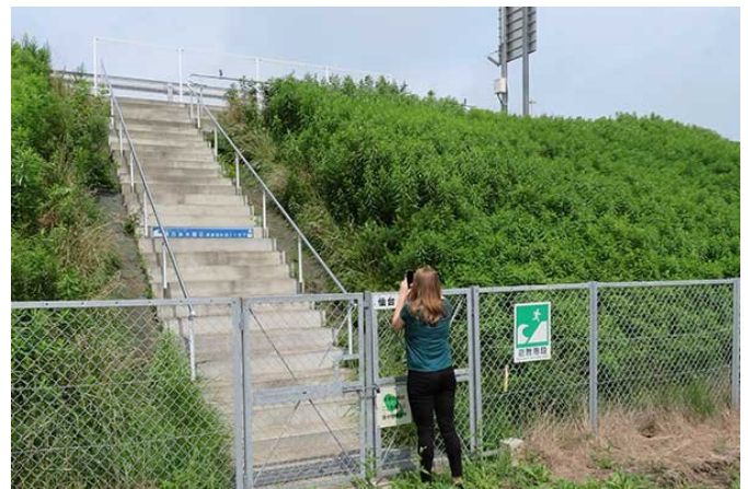
The Sendai-Tobu Road evacuation stairs, which played a role in holding back the 2011 tsunami. As a result, construction of evacuation stairs in and around the city of Sendai has proliferated Credit: Tohoku University
