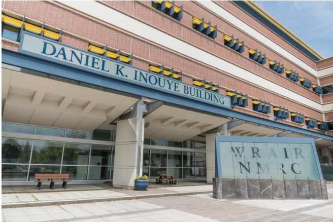
The Daniel K. Inouye building on the Walter Reed Army Institute of Research campus. Credit: WRAIR
